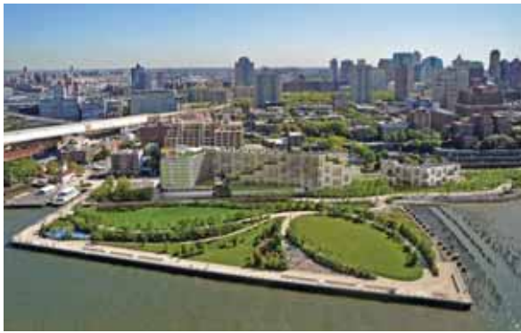
Rogers Marvel has designed a 550,000-square-foot building that steps back from the Michael Van Valkenburgh-designed Brooklyn Bridge Park.
